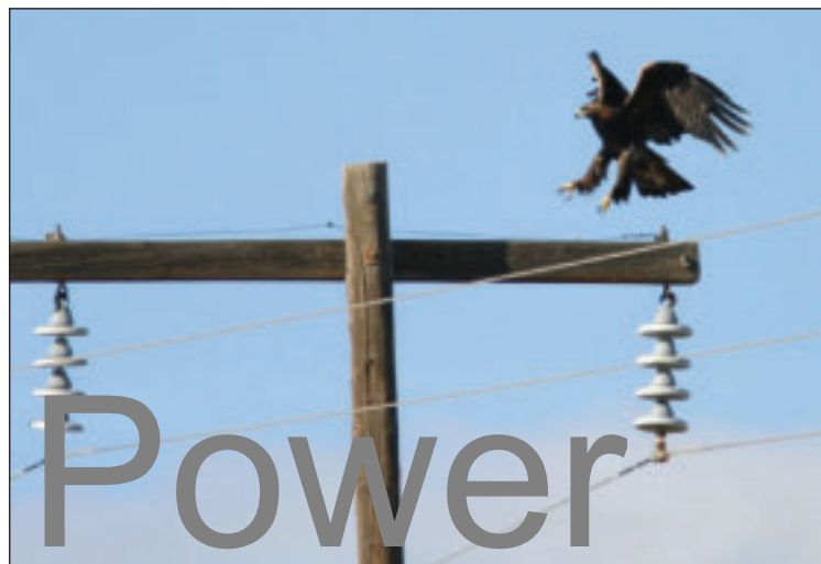
FIGURE 2.2: Golden eagle landing on avian-safe pole. Early research on avian electrocutions and pole modifications focused largely on golden eagles.
