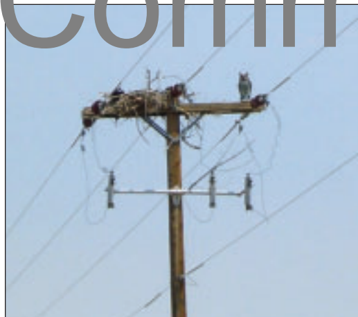
FIGURE 6.26: Osprey nest constructed on pole with plastic owl intended to haze birds.
