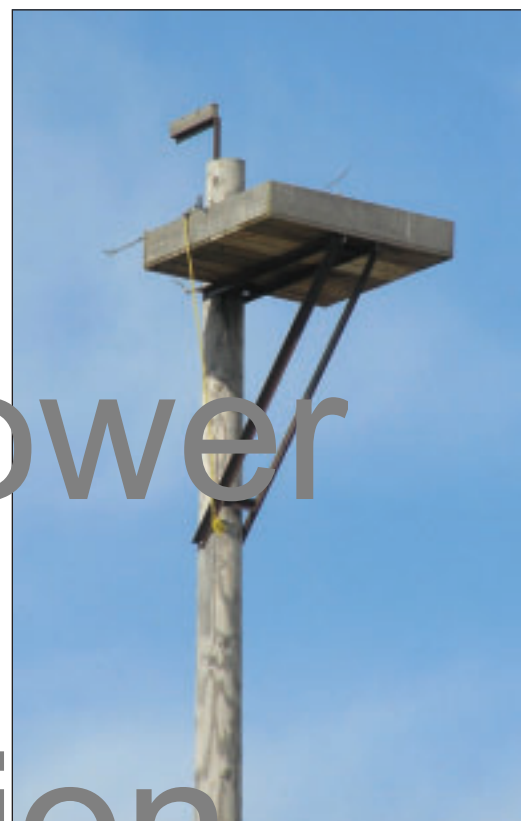
FIGURE 6.14: A simple and cost-effective nesting platform built for ospreys in Washington. Pallets can be used as platforms, providing ospreys with a flat resting area.
