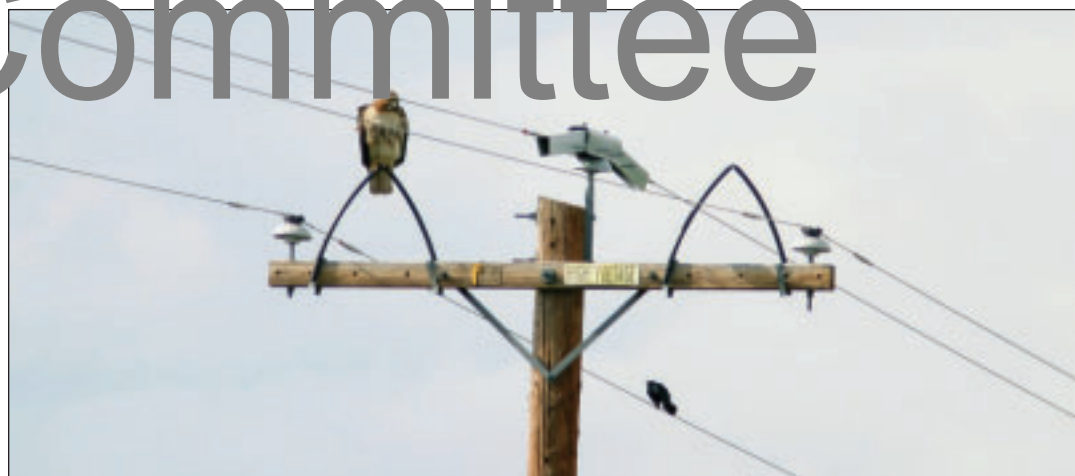
FIGURE 2.5: Perch discouragers have been installed on utility poles to prevent raptors or corvids from preying upon sensitive species. However, this is not recommended, as perch discouragers are intended to manage where birds perch, not to entirely prevent perching.
