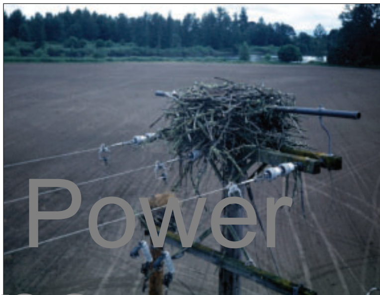
FIGURE 6.23: A segment of plastic pipe was installed on a dead-end pole in Oregon to discourage osprey nesting. However, the osprey pair continued nest construction after the pipe was installed.
